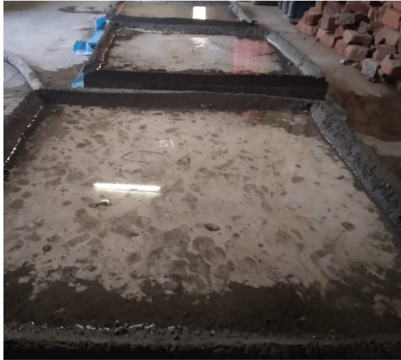
Fig 4: Curing of slabs
